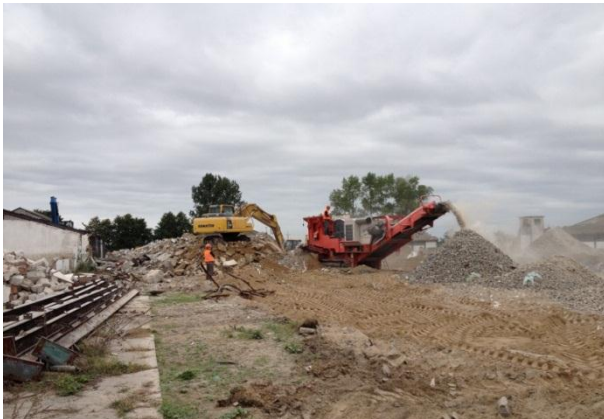
Farm base refurbishment
