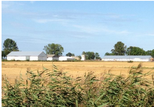
After farm base refurbishment
