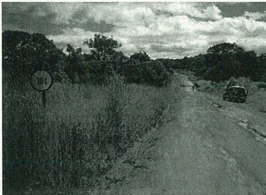
Source: Photo by JICA Study Team Photo 15.1.2. Weight Limit for Bridge (R658)
