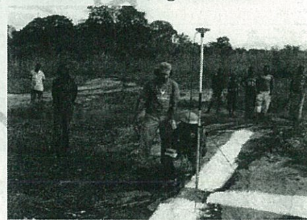
Photo A.1.1 Signalization
